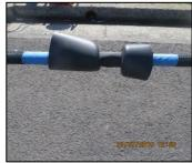
Centrally position Shrink Sleeve, heat from centre then out with Heat Gun.
