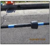
Shrink the other end until firmly shrunken onto the strop.
